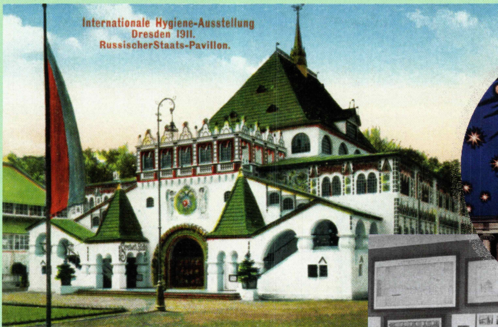
Above: The Russian Hygiene building at the Dresden Exhibition. Designed by architects from its mother country.
